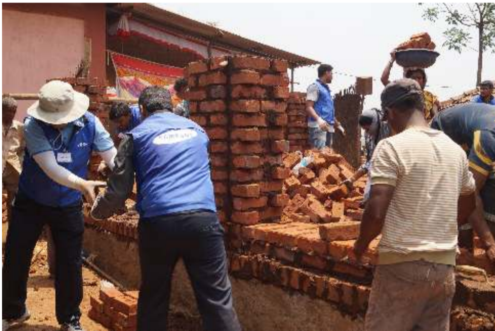
Volunteers at House Construction at Laval village, Ambernath.
