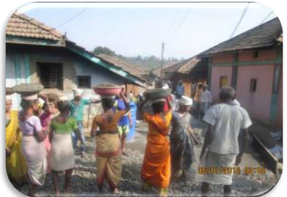
Road construction by SHG members at Kuderan
